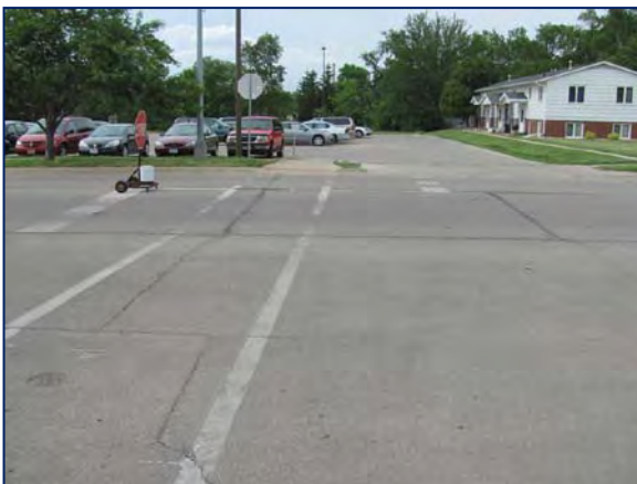
The existing crosswalk on Seerley Boulevard includes a roll-out STOP sign. The crosswalk does not include school crossing assemblies.
