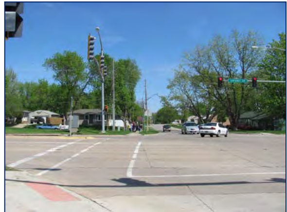
Traffic signal at Katoski Drive and Downing Avenue intersection. This intersection is the main entrance to the school and the location most pedestrians use to exit the school grounds. There are no pedestrian signal heads on the east leg of the intersection.
