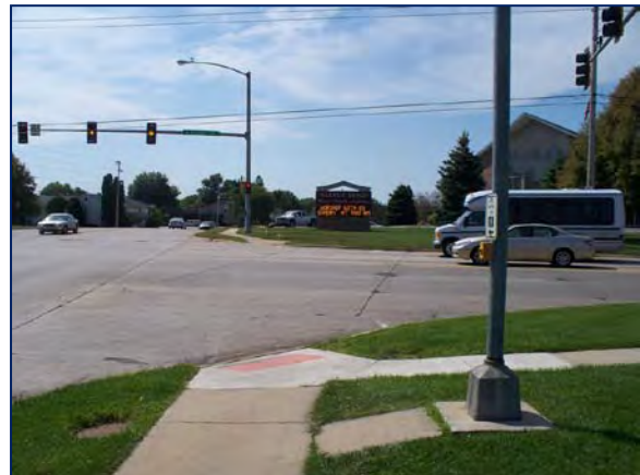
Traffic signal at Ansborough Avenue and Ridgeway Avenue. Push-button pedestrian signals are located on the west and south legs of the intersection. The pedestrian signals on the south side of the intersection do not lead to any sidewalk on the east side of Ansborough Avenue or the south side of Ridgeway Avenue.
