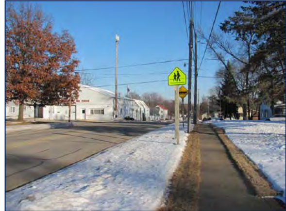
The school crosswalk on 14th Avenue at 4th Street. The actual sign location for the crossing on the west side of the crosswalk is 50 feet away. 14th Avenue is the main entrance into Gilbertville from the west. This is County Road D38. The speed limit on 14th Avenue is 25 mph. Up-to-date MUTCD signing is needed at this crosswalk as well.
