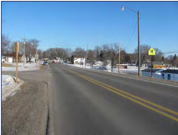
The school crosswalk on 20th Avenue has no sidewalks leading to it. The speed limit on 20th Avenue is 35 mph. The existing signing does not meet the latest standards as stipulated by the Manual on Uniform Traffic Control Devices.
