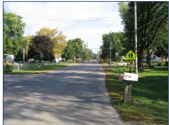
Looking north on Grand Boulevard at Central Avenue intersection. The existing pavement is 26 feet wide which is too narrow for pedestrians and vehicular traffic particularly in the winter.
