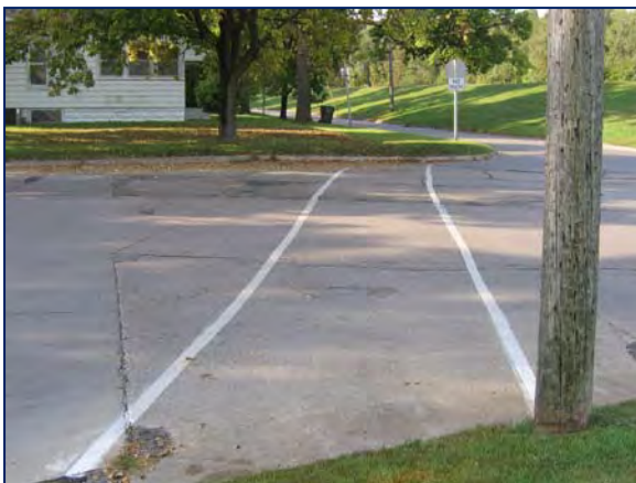
These photos show the intersection which lacks proper crossing signing and traffic control. The westbound vehicle along Parker Street does not have a STOP or YIELD sign.
