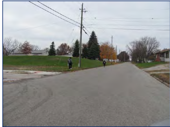
Students walk in the street along Louise Street due to a lack of sidewalk.
