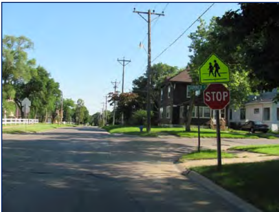
Looking south toward the Sumner Street and Mobile Street intersection. The MUTCD states that a school crossing assembly shall not be installed on approaches controlled by a STOP sign.
