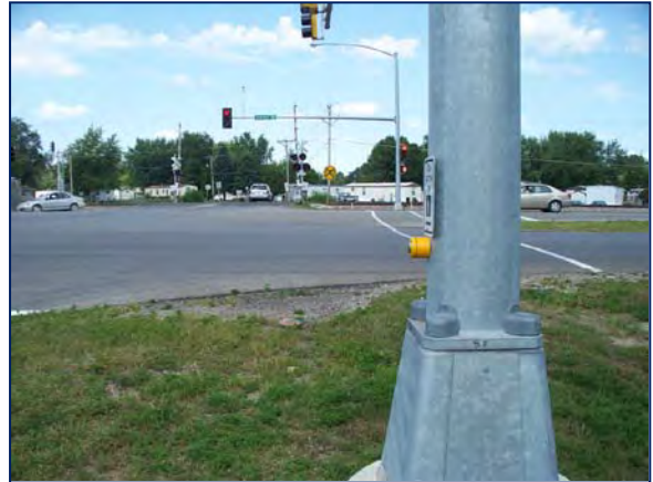
The existing Dubuque Road school crosswalk at Adrian Street/Idaho Street intersection does not have sidewalk crossing the railroad tracks or up to the intersection. The traffic signals do not have sidewalk to access the push-button actuators.
