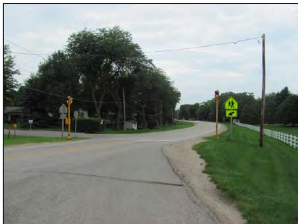
The IA 58 pedestrian signal and school crosswalk are located between Sunset Drive and School Street. There is no sidewalk on either side of the crosswalk.
