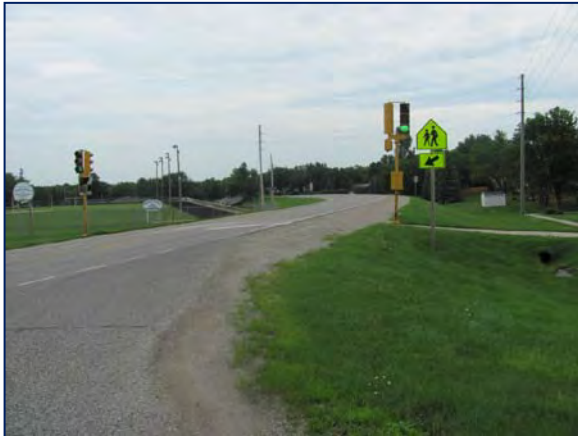
Pedestrian signal and school crosswalk are well designated with current signing and pavement markings.
