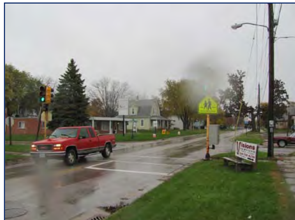
Signalized pedestrian crossing at Magnolia Parkway and Falls Avenue.
